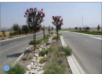
Median bioswale with dry river bed
