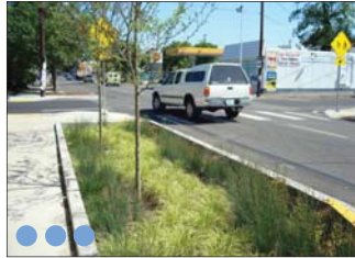
Sunken bioswale with curbed edge
