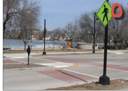
Decorative crosswalk border w/ RRFBs
