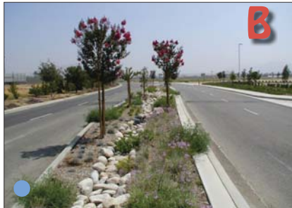
Median bioswale with dry river bed
