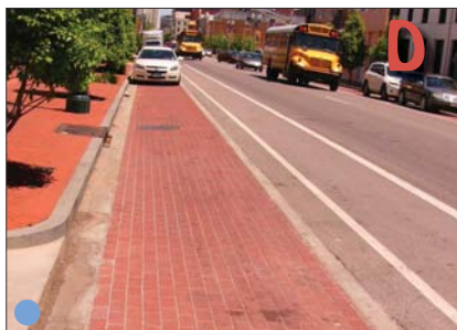
Permeable pavers in parking lane
