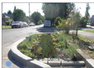
Bump out bioswale
