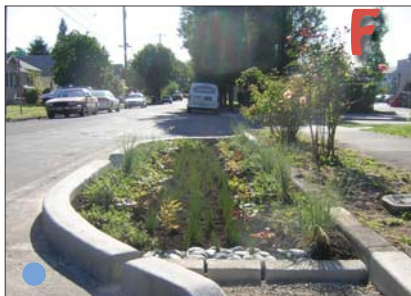
Bump out bioswale
