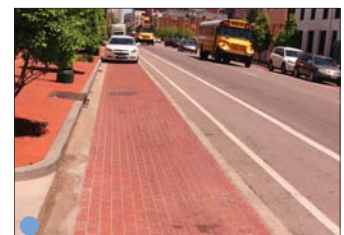
Permeable pavers in parking lane
