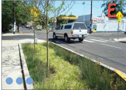
Sunken bioswale with curbed edge
