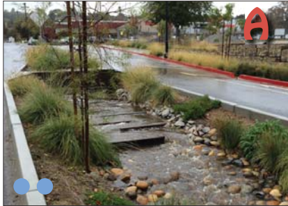
Median bioswale with dry river bed
