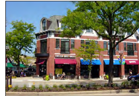
Corner building with attractive details such as decorated cornices, cast-iron balcony railings, dormers, and signs incorporated into sign bands.
