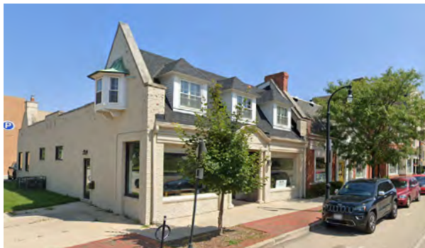
Traditional storefront building with characteristics of a Commercial House.
