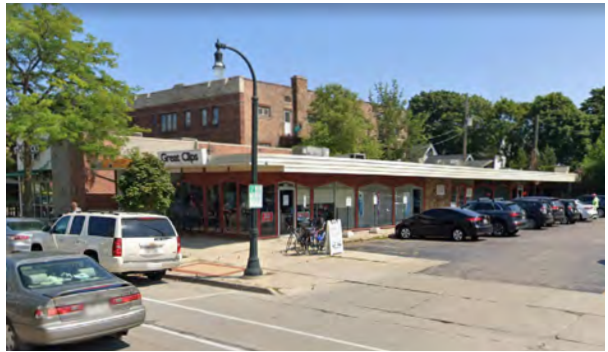
Single-use, single-story buildings and strip centers.
