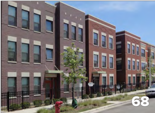
Poor fencing style, not connection to street, building feels like a large wall, too long
