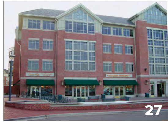
Positive, awning, window details, irregular roof
