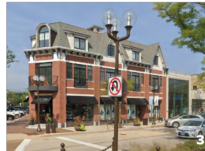
3 Balcony, good angles, color, materials, work well w/ Shorewood Breaking down the scale with roof, Good height, not gimmicky, dormers pastiche, Like this style top floor windows Positive, materials, roof line, inviting, trees
