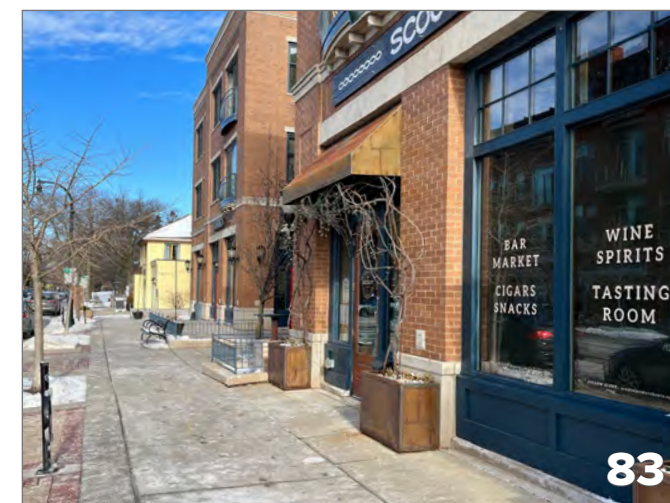
83 Wine shop deck, Banded? courtyard/eating area, great space for walking, multiple uses for courtyard Mix of materials, color, interest, planters
