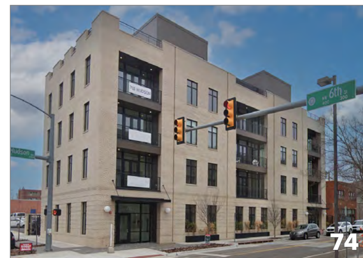
74 Like green spaces and ground level balconies Too much concrete, no joy, all windows too similar Too hard on ground floor, not enough articulation Cold, hard, neutral, doesn't scream anything
