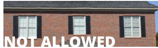
Inappropriately Sized Shutters.
