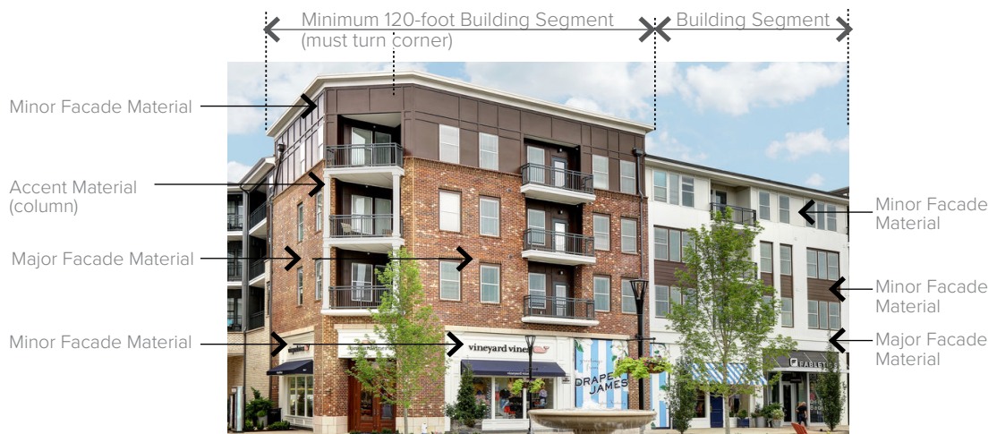
Figure 2-1. Example of Major and Minor Materials on a Facade
