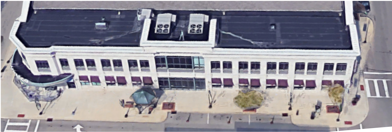
Figure 2-R. Rooftop Utilities Screened from the Public Way by a Parapet
