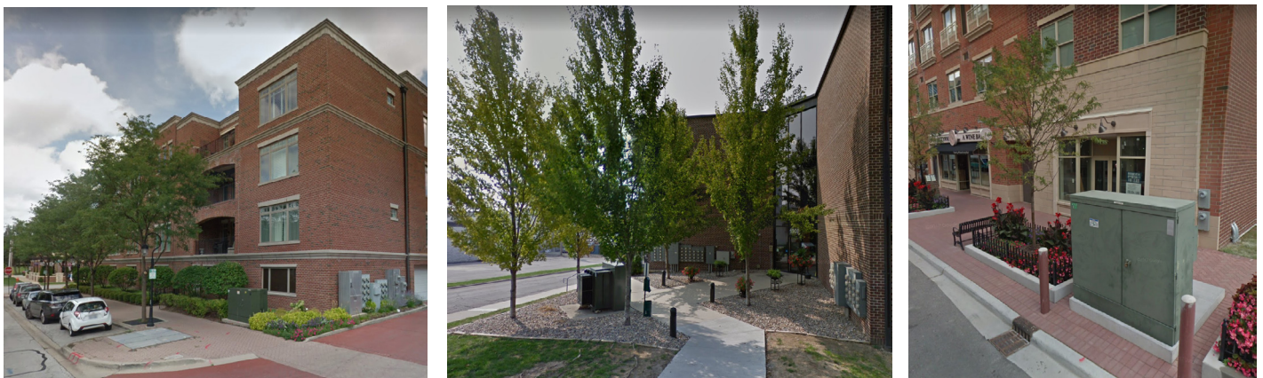
Figure 2-T. Examples of Poorly Located Utility Appurtenances on Primary Streets
