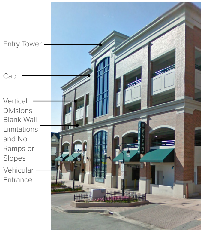
Figure 2-Q. Example of a Parking Structure
