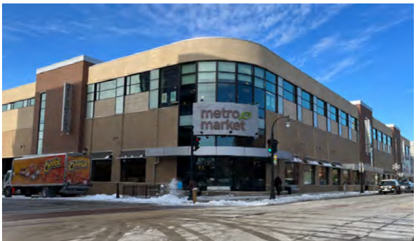
Redevelopment of the PicknSave, Walgreens, & large surface parking lots into a new grocery store, mixed-use buildings, and structured parking.
