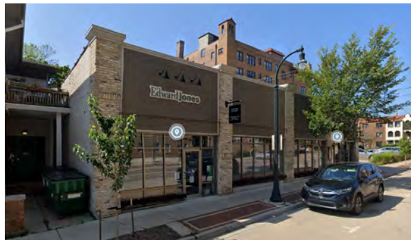
Single-use storefront building just east of Farwell.
